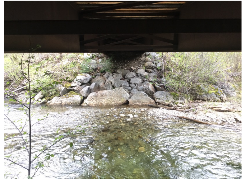
Right Bank Abutment when facing downstream
