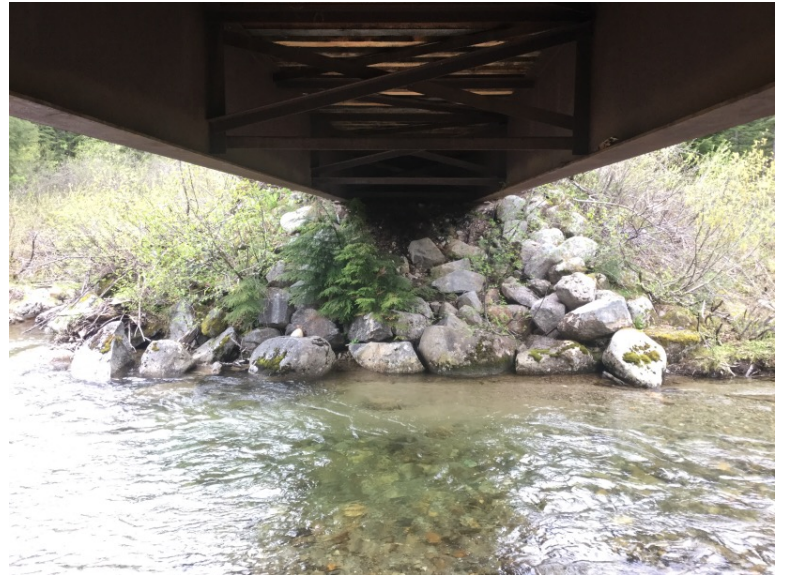
Left Bank Abutment when facing downstream
