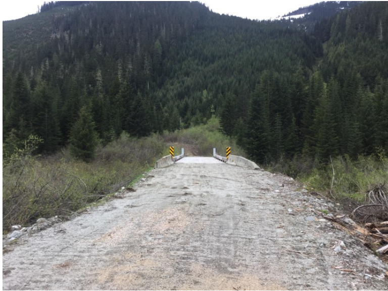
Approach from Right Bank when facing downstream
